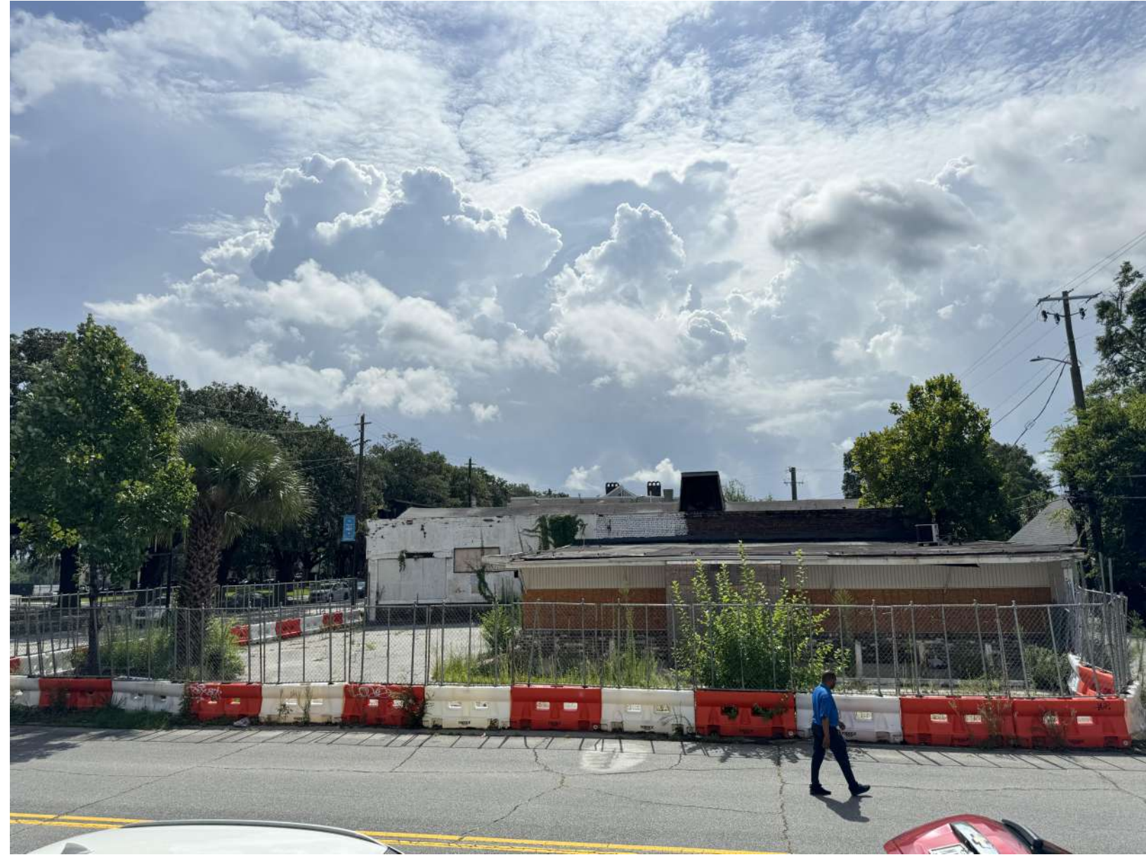
4 EXISTING SITE CONTEXT PHOTO - HABERSHAM ST. HDRB 0.2
