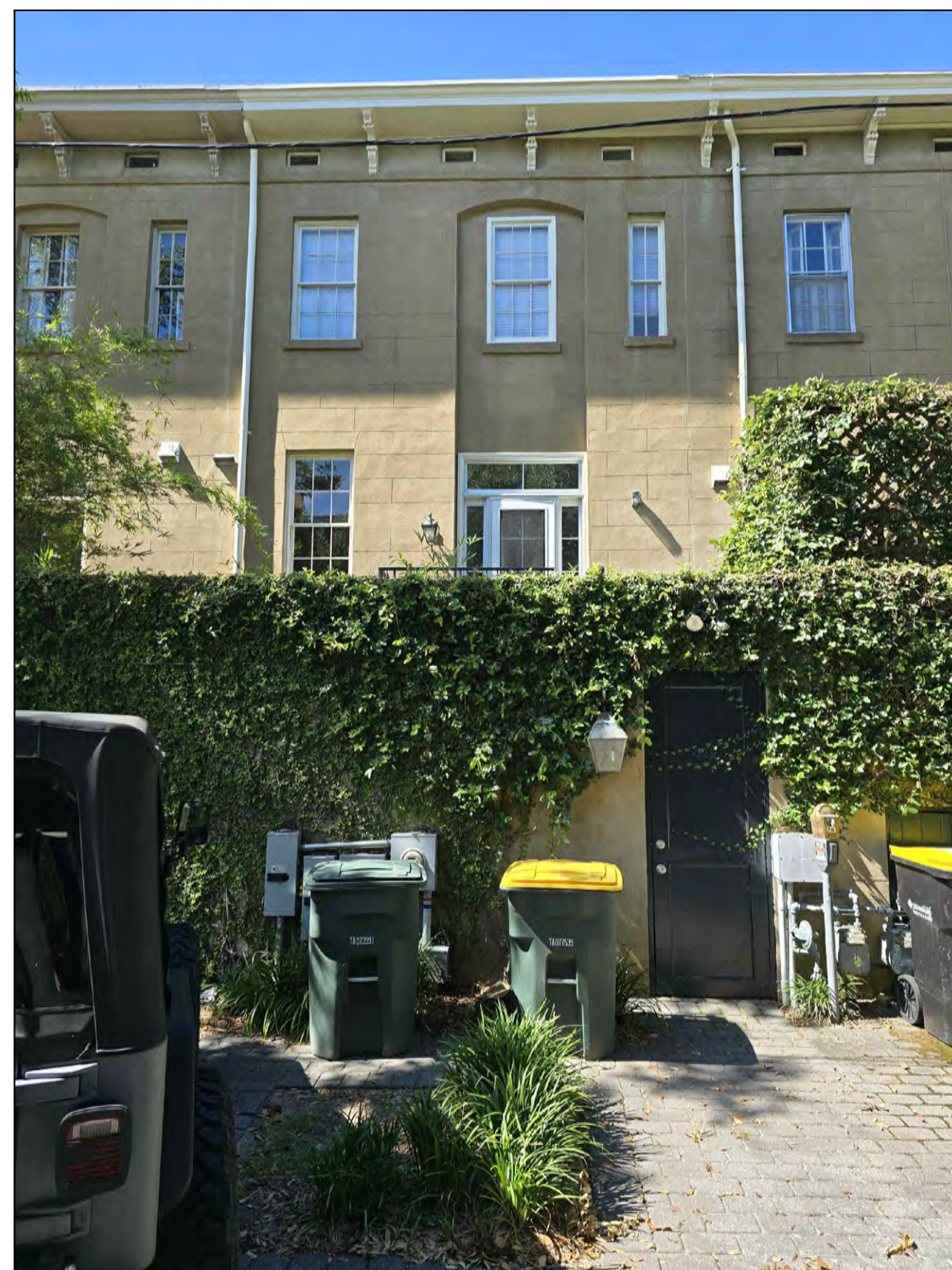
REAR FACADE FROM EAST MACON STREET
