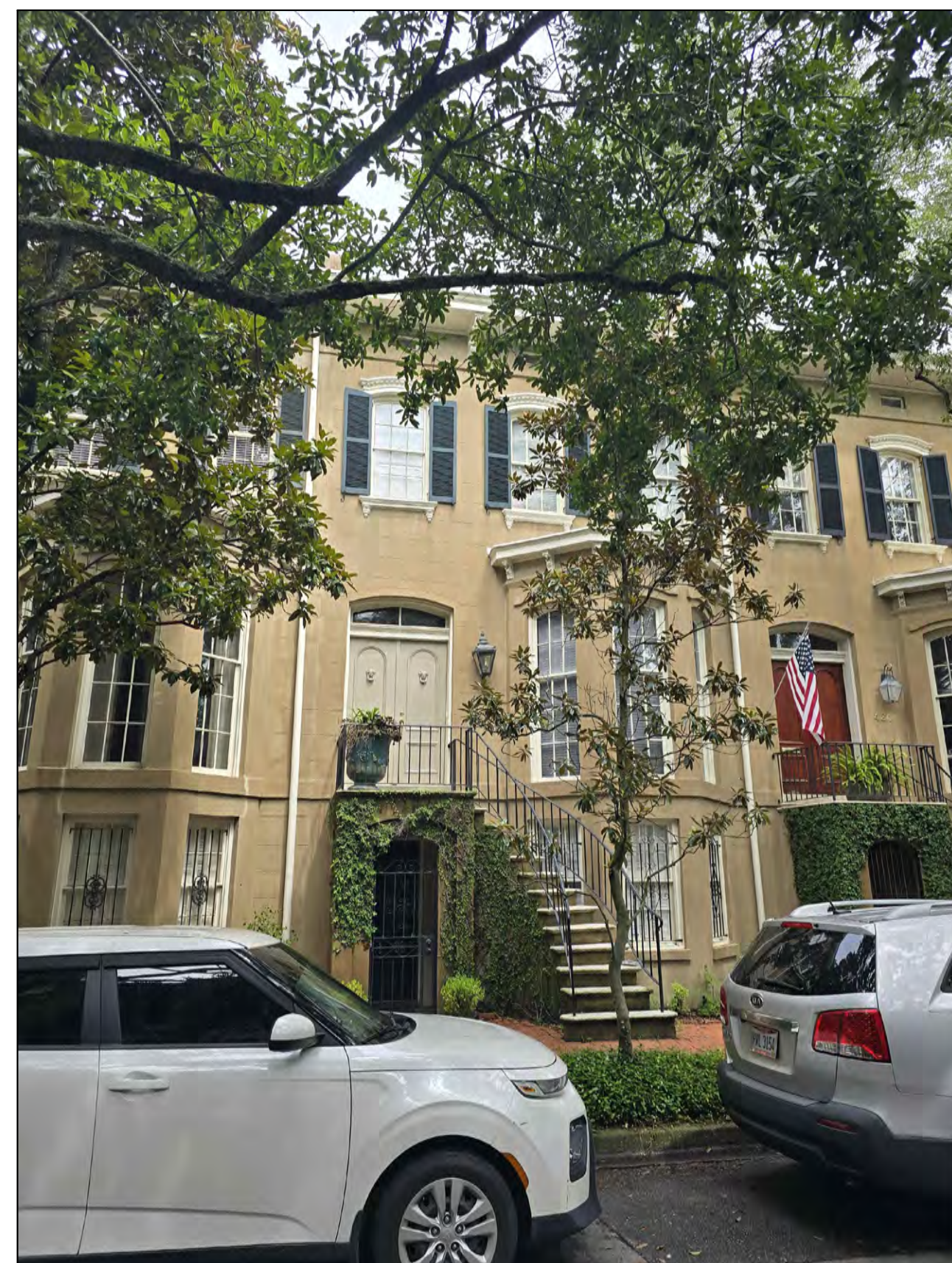
FRONT FACADE EAST CHARLTON STREET
