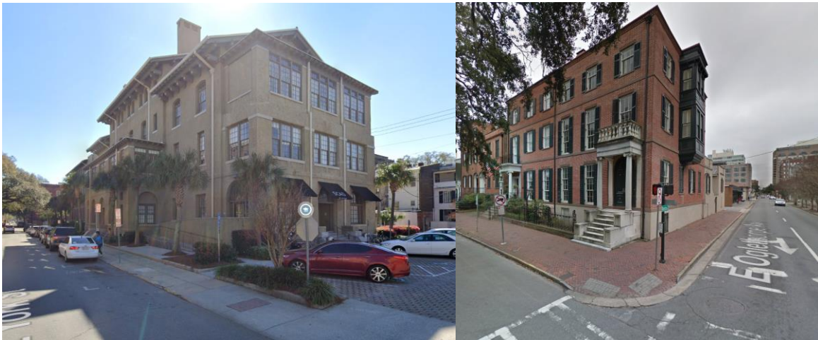
Figure 5 – 115 East York Street & 101-109 East Oglethorpe Avenue
