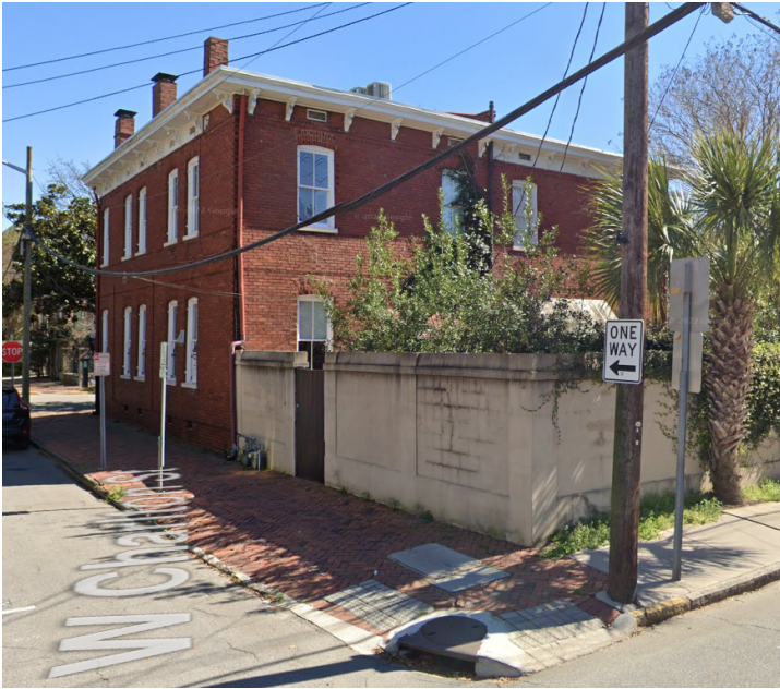
REAR FACADE - March 2022
