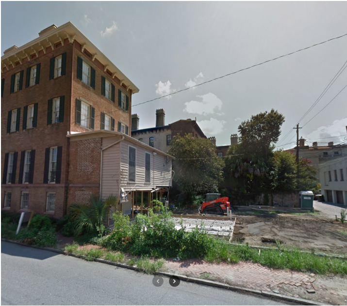
REAR FACADE - August 2017
