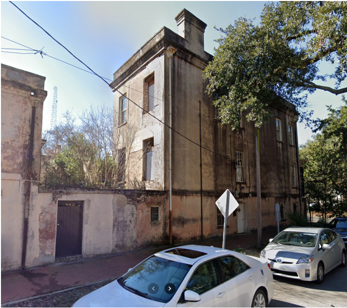
REAR FACADE - JANUARY 2019
