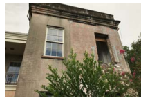
PHOTO 8 (HOSTING OF FORMER ADDITION)
