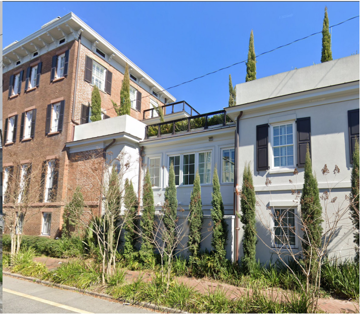
REAR FACADE - MARCH 2022
