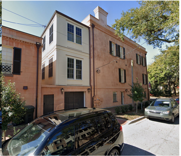
REAR FACADE - MARCH 2022
