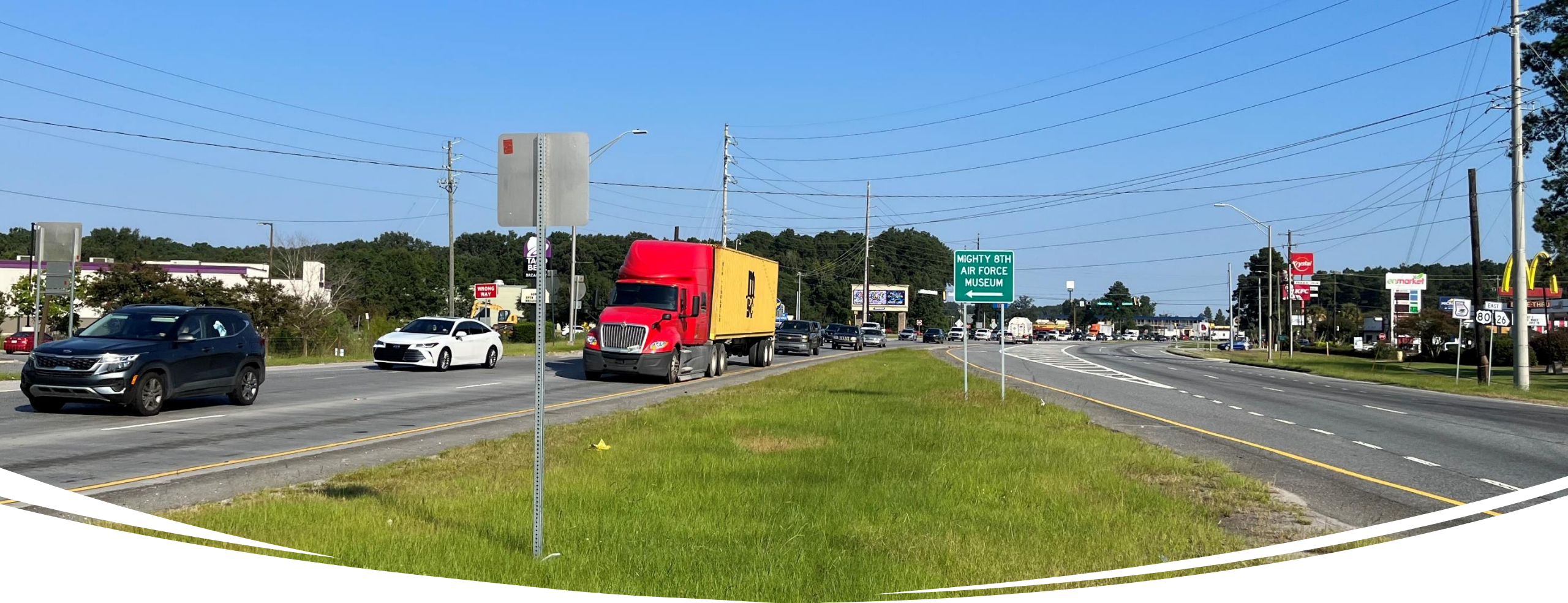
Westbound SR 26/US 80 east of I-95 Northbound Ramps
