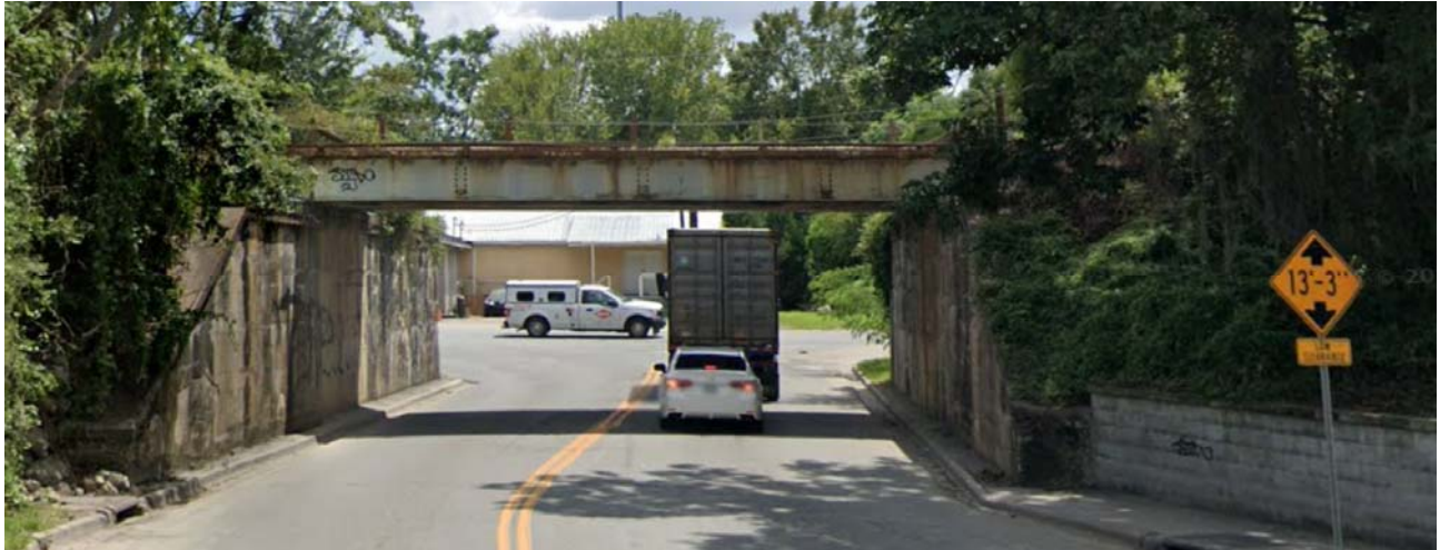
FIGURE 3.4 VERTICAL CLEARANCE AT E. LATHROP AVENUE
