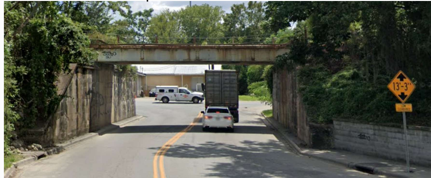
E. Lathrop Ave. north of Louisville Rd.
